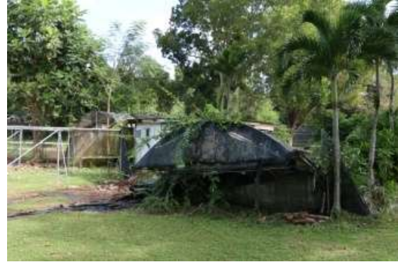
Figure 2: Damages caused by Hurricanes Irma and Maria are still visible at the nursery. Arecibo, Puerto Rico. USDA Forest Service photo.
