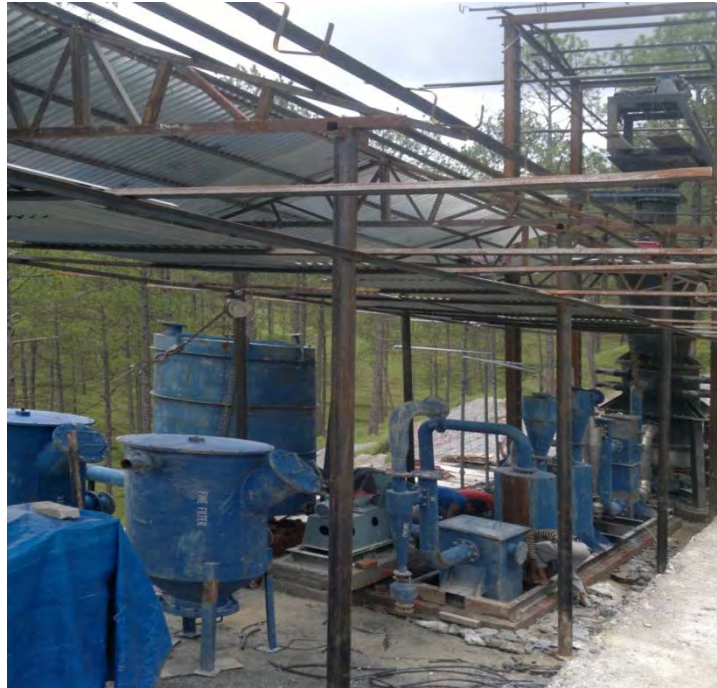
Pine needle gasifier under construction
