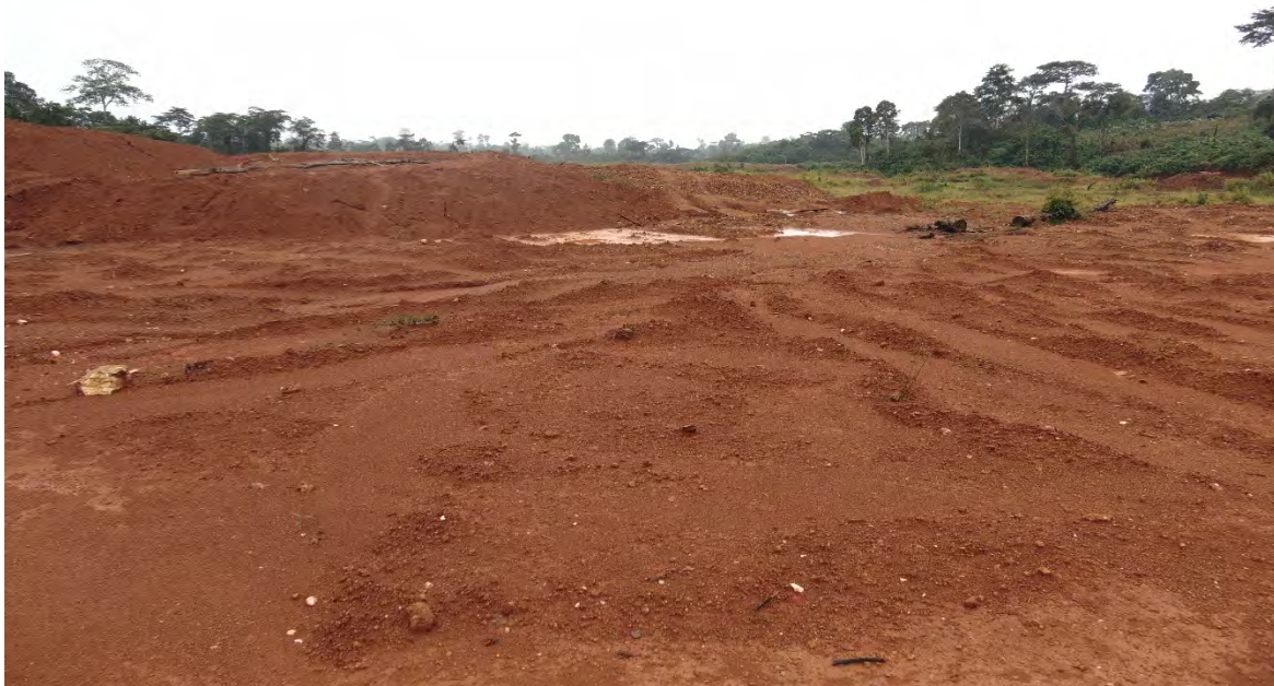
Picture 9: Cleared land cover of some part of the TOFR
