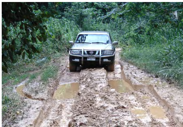
Picture 1: Jolting road connecting the adjacent communities and TOFR
